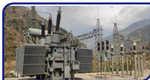
POWER TRANSFORMER AT INTERCONNECTING SUBSTATION END
